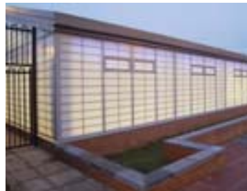
Hemsworth Managed Offices Hemsworth, Yorkshire, UK Architect: Atkins Architects; Photo: David Jewel
